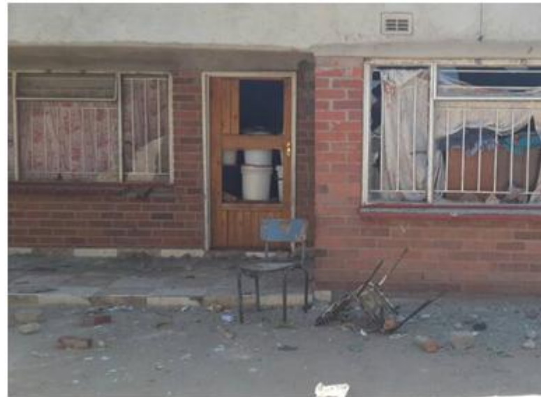
Property damaged during the attacks
