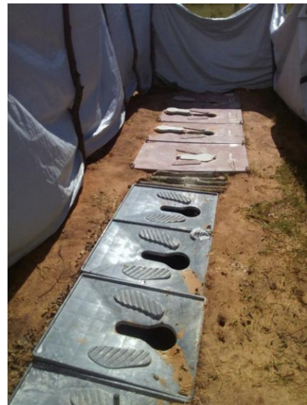
Figure 2: Toilets at the camp, ZPP photos
