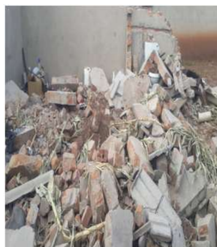
Some of the structures destroyed in Arcadia Harare
