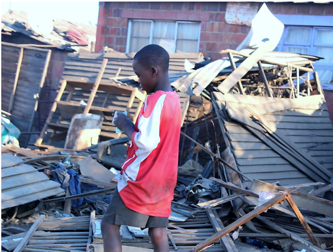
A boy walks past the remains of a tuckshop that was demolished in Highfields, Harare. The tuckshop also served as a house for the owner and is one of the many informal trading spaces and houses demolished under an operation by the Zimbabwean government in June 2021.
